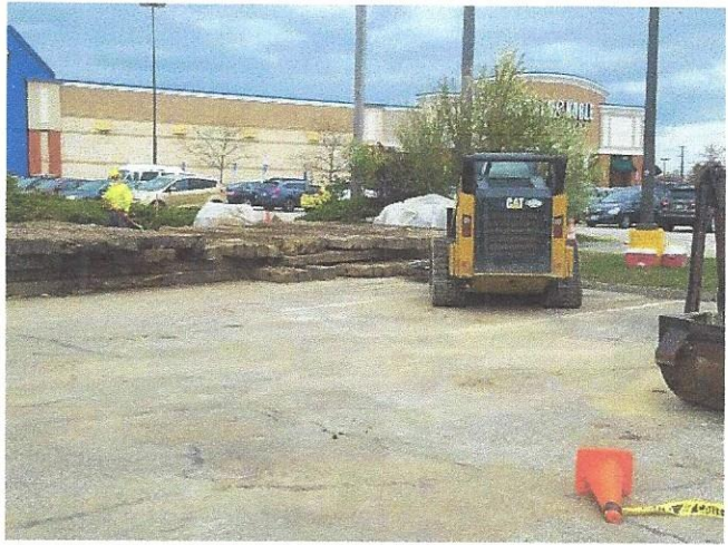
Fig 2: Timber matting used to elevate equipment, viewing north.
